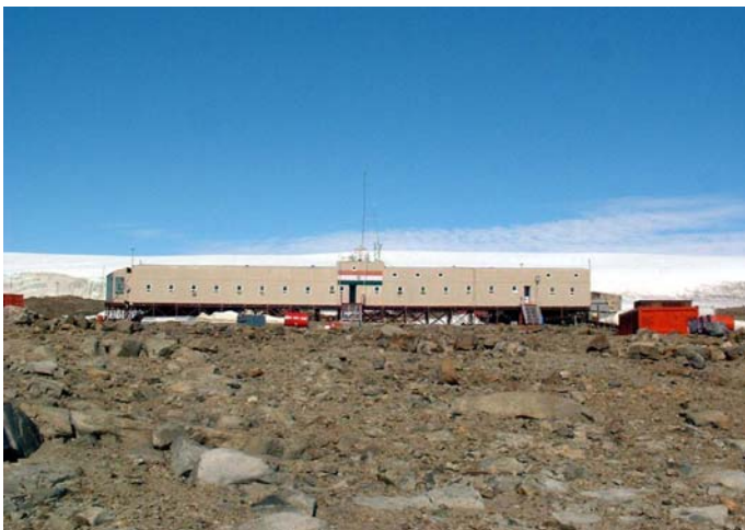
Close-up front view of Maitri station
